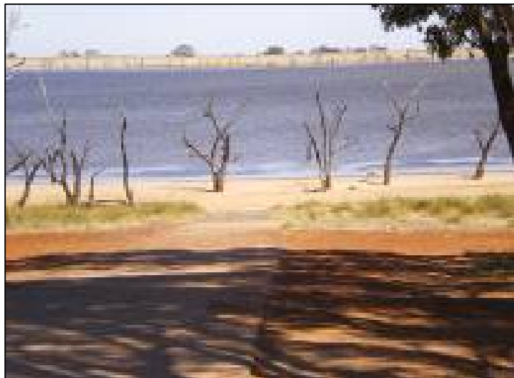
Photo 9: Existing boat ramp
